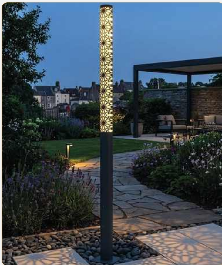
D-SLS-03 in service — existing shaft retained
